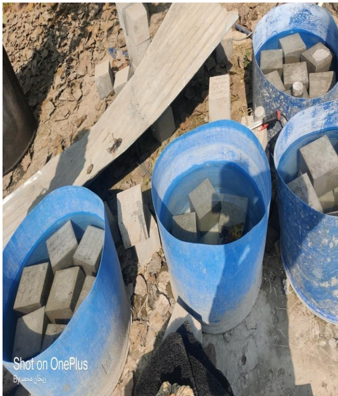
Fig. 3 Curing of concrete
