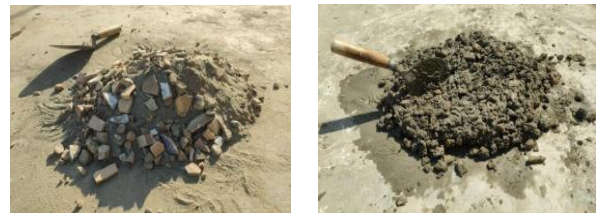
Fig.6- Mixing of Material
