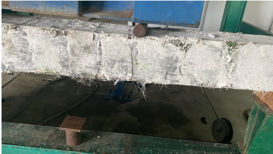
Fig 4.3.3: Cracked beams after retrofitting
