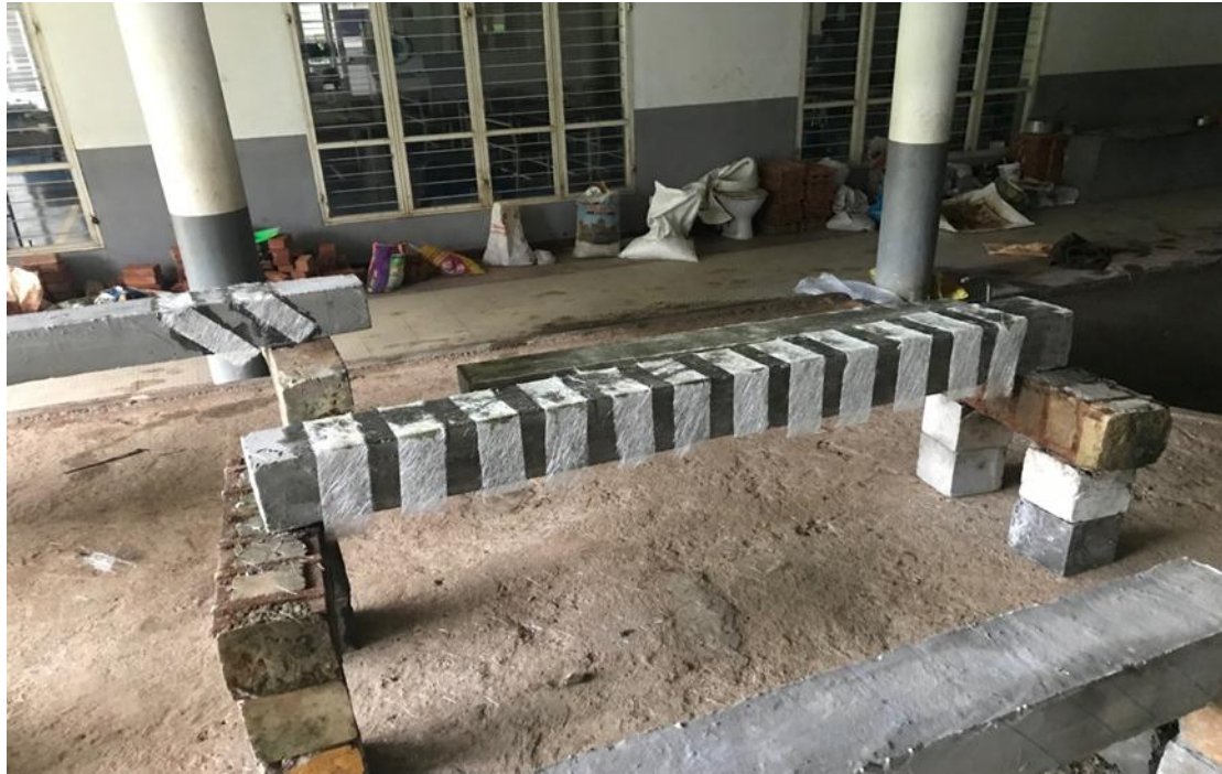
Fig 3.3: 90 degree wrapping using glass fiber sheets
