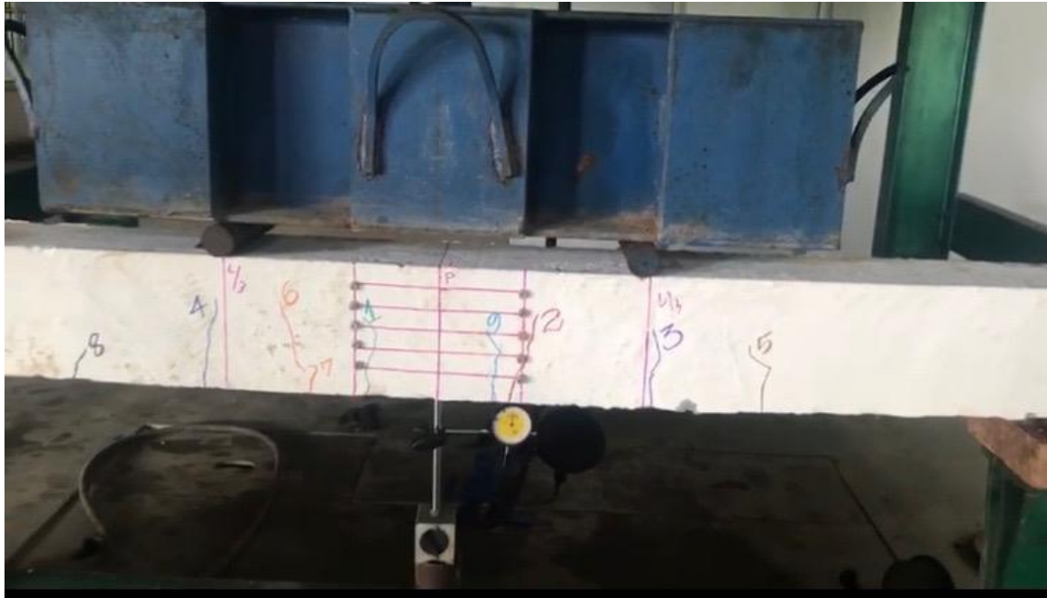
Fig 4.3.2: Cracked specimen marked
