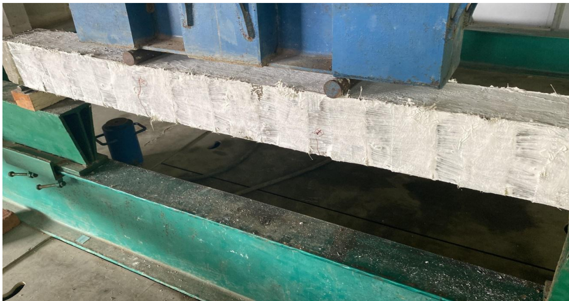
Fig 4.4.1: 90 degree strip wrapped collapsed beam for retrofitting
