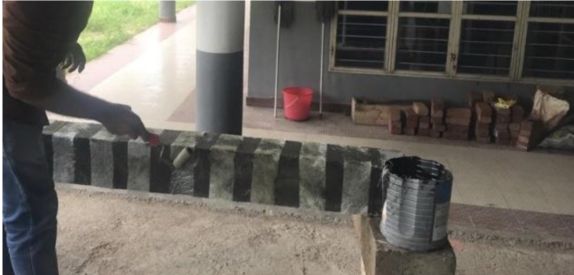
Fig 3.1: Application and fixing of glass fibre sheet and resin mortar
