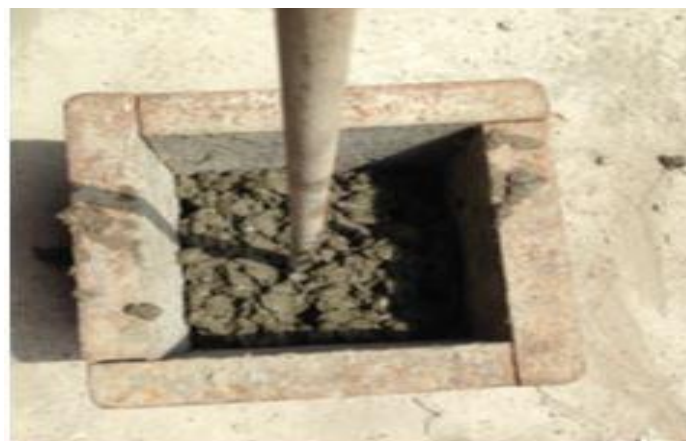
Fig -3: Rodding of pervious concrete
