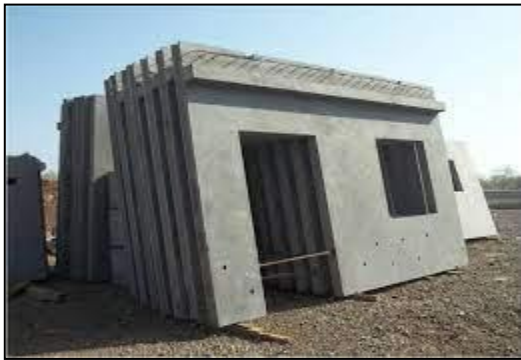
Fig. No. 6 Prefabricated walls
