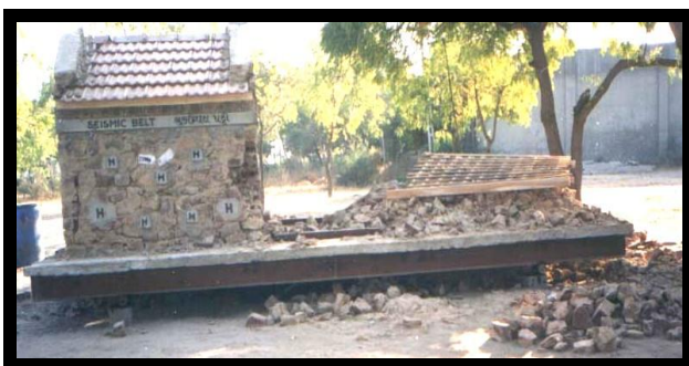
Fig-8: Stable / slightly damaged improvised model v/s total collapsed Traditional Model
