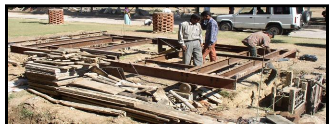
Fig-2: Table Frame Erection
