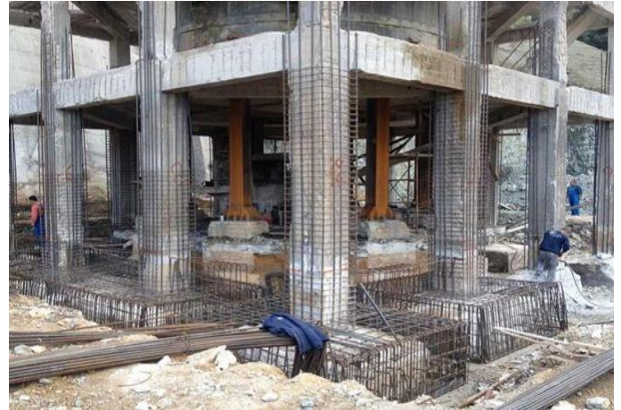
Fig -1: Retrofitting of the structure
