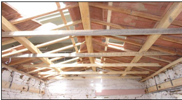
Fig-5: Wooden in-plane Bracing
