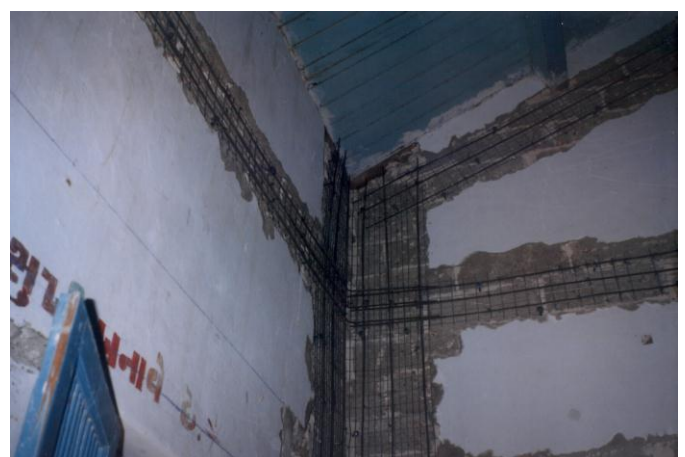
Fig-4: Corner belt with vertical reinforcement
