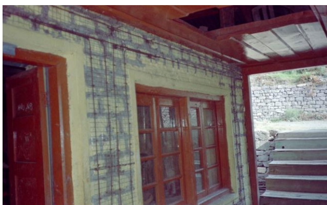
Fig-2: Horizontal and Vertical Seismic Belts
