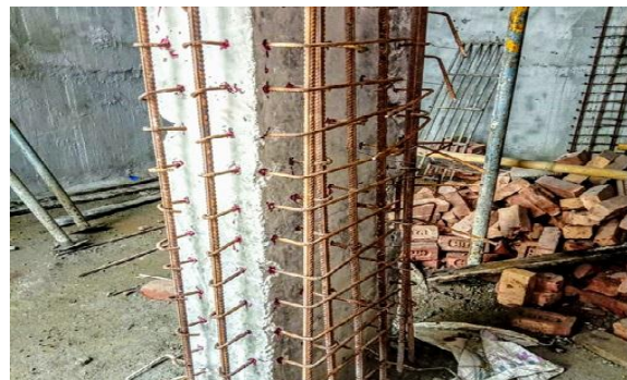
Fig Retrofitting of column
