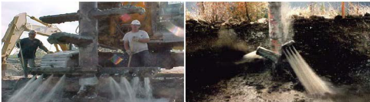
Figure 3: Parts of wet mixing tool showing injection of slurry into the soil (Porbaha et al, 2005)
