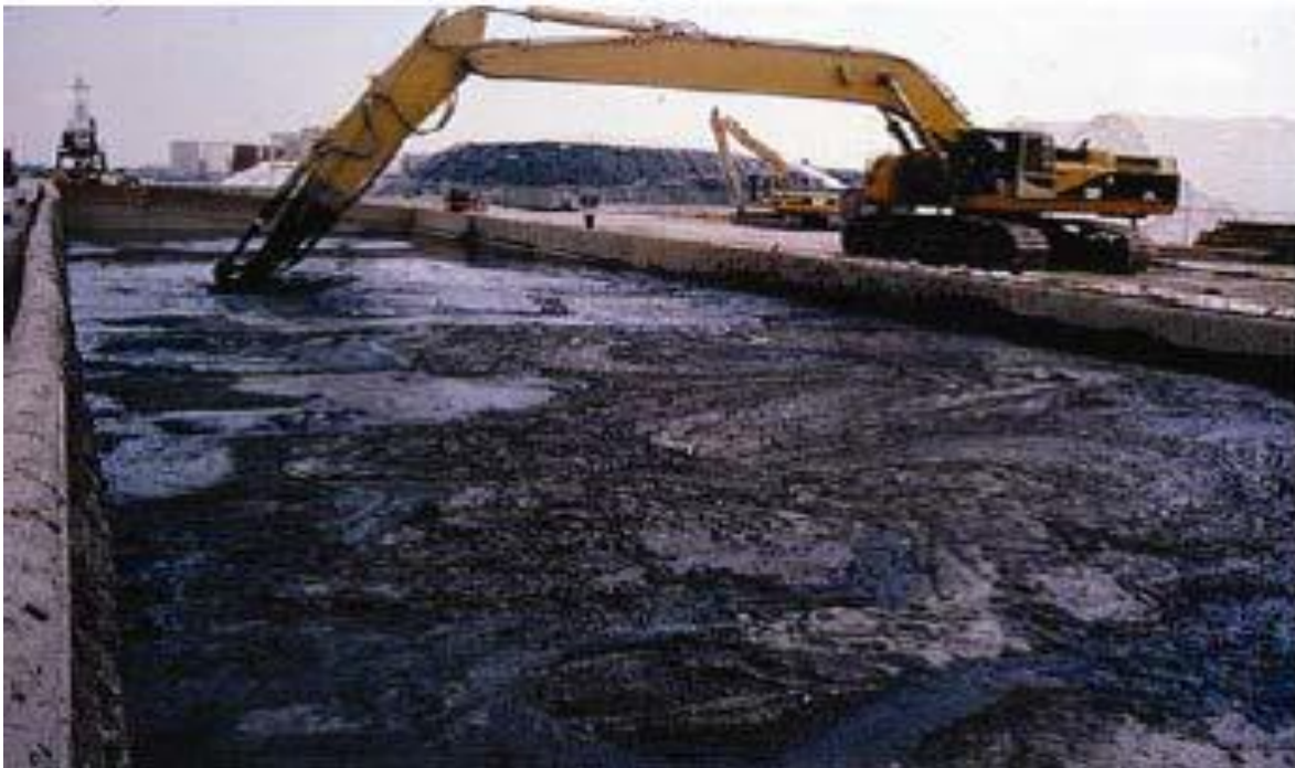
Figure7: Ex-situ for on-site use stabilization (mixing in place of contaminated dredged materials) (Wiki, unpublished document)
