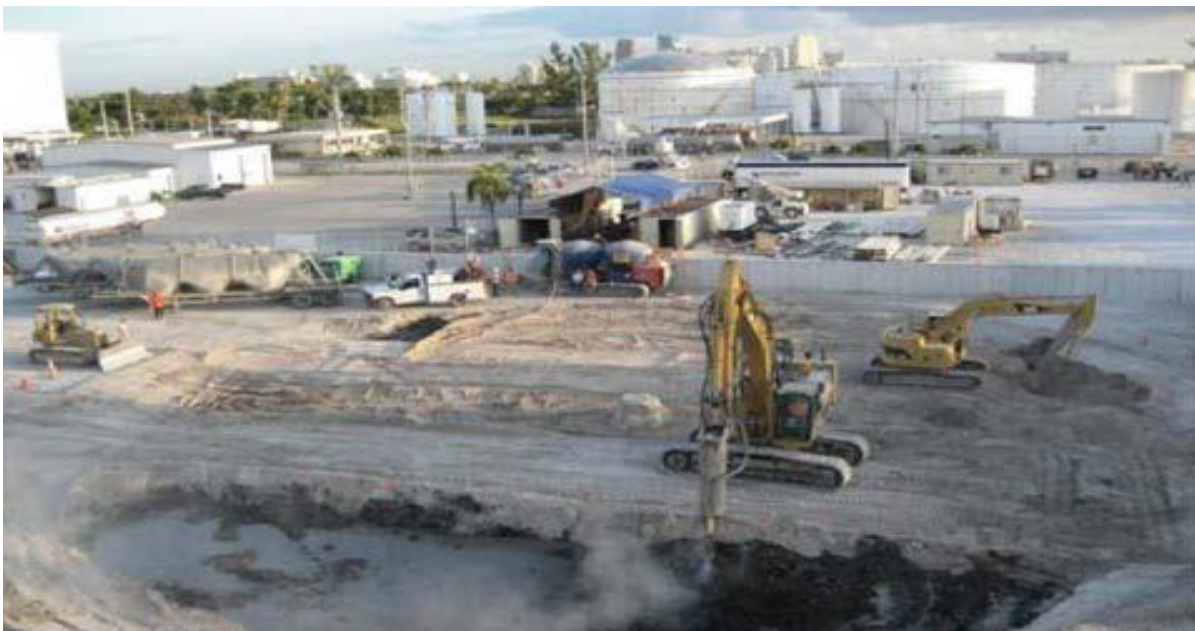
Figure 6: Mass stabilisation with dry soil mixing of soft wet organics was used to manage settlement for storage tanks at Port Everglades, Florida, (Hayward Baker Inc.)
