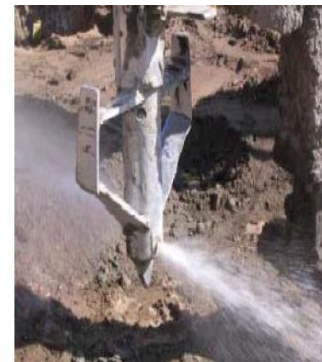
Figure 5: Nordic modified dry mixing tool (Larsson, 2005)
