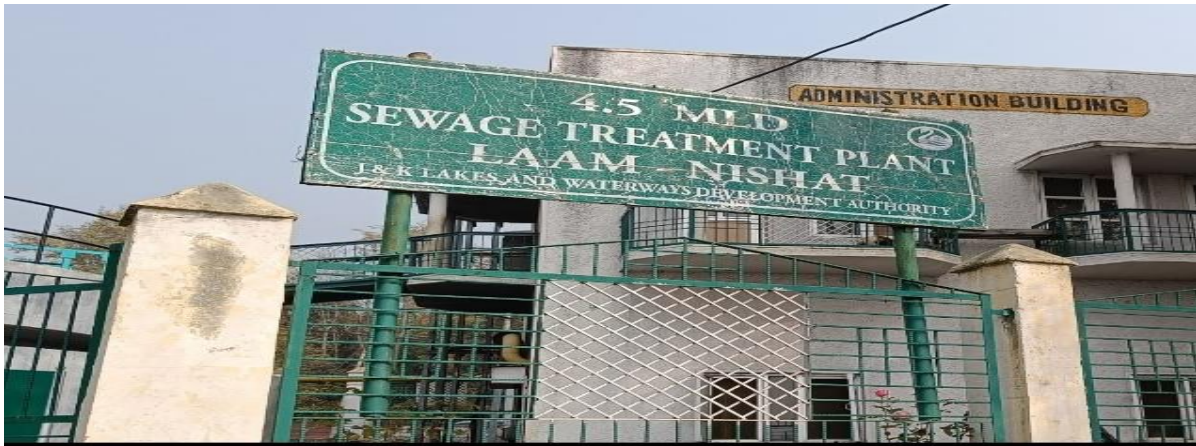
Fig-1: Showing STP Nishat (FAB)
