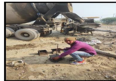
Figure-2 Cube Casting
