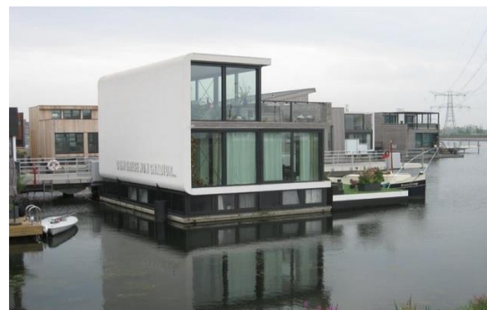
Fig- 1: Floating Houses in Iburg, Amsterdam, Netherlands
