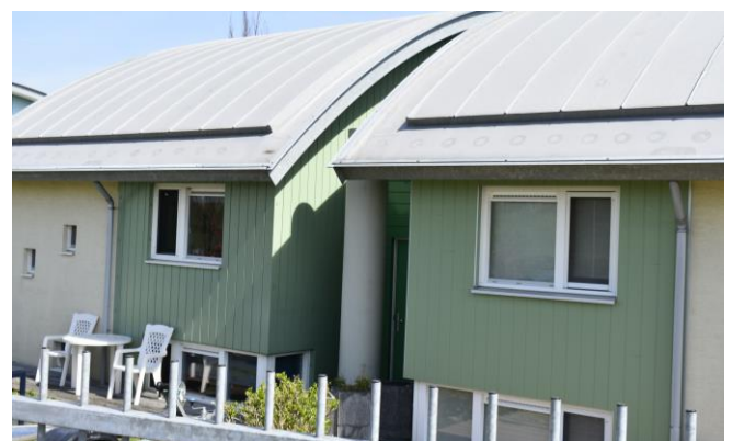
Fig -4: The guidance post between the two units of amphibious houses at Maasbommel, the Netherlands (Original photo shot by the second author)
