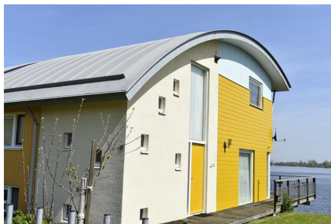
Fig -2: Amphibious house during dry condition on the banks of Maas River at Maasbommel, the Netherlands (Original photo shot by the second author)
