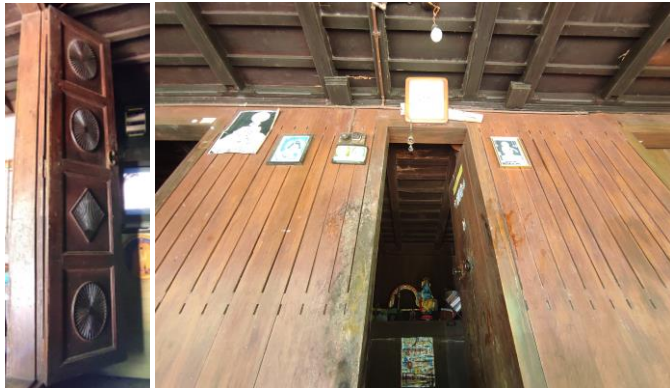
Fig -8: A wooden door with detailed wooden carvings(left) and wooden walls and roof with the old 'ara' converted into a 'pooja' (religious) room of Thevarpathiyil home (right) (Original photos shot by the first author)
