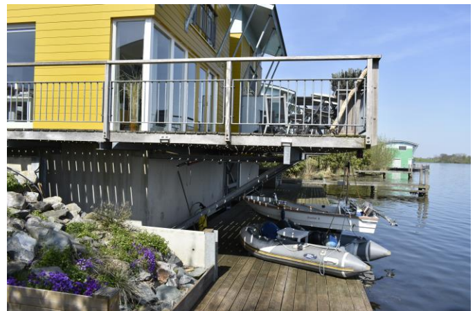
Fig -3: An amphibious house and a fully-floating house built near and in Maas River at Maasbommel, the Netherlands (Original photo shot by the first author)
