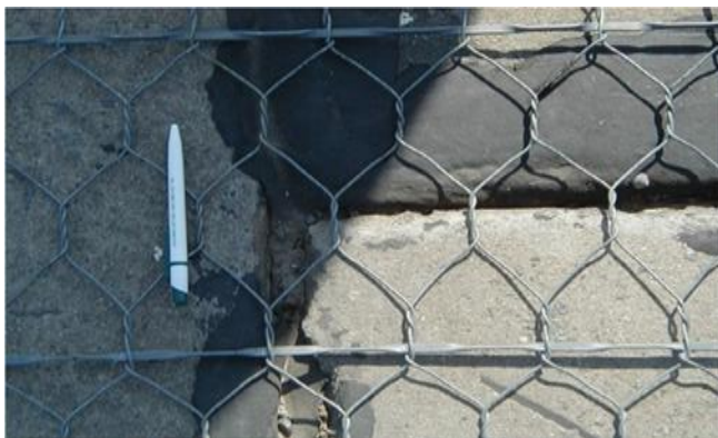
Fig 2 Steel reinforcement mesh
