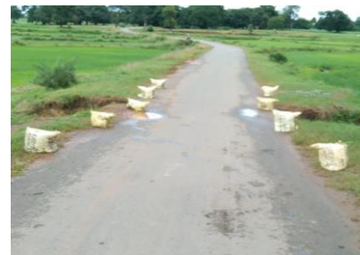
Figure 3: Unsafe barricading
