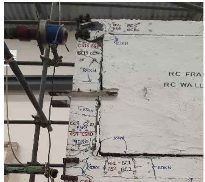
Fig -15: Debonding of wall panel
