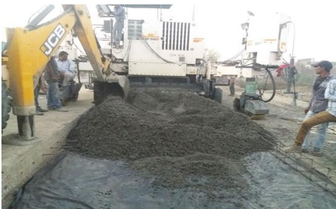
Fig No 2. Placement of Concrete
