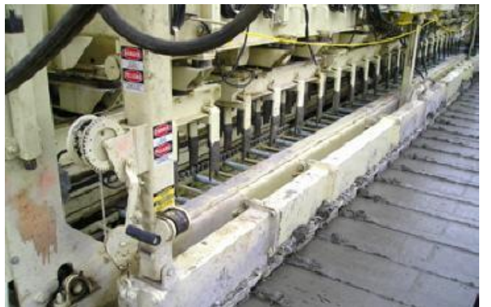
Fig No 4. Placement of Dowel Bars in Concrete Slab
