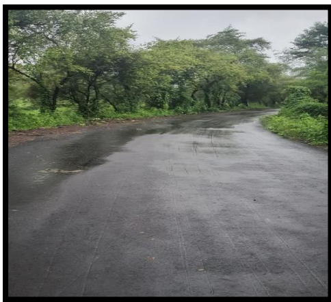
Figure -3: Bitumen Road
