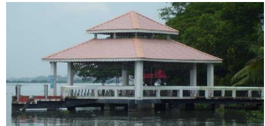
Fig -2: Boat Jetties along Marine Drive
