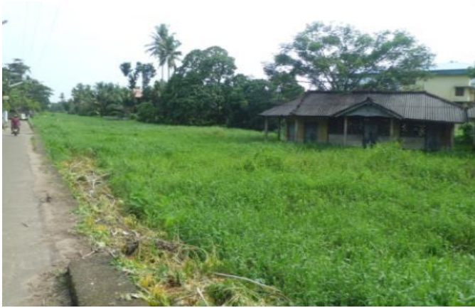
Fig -1: The dilapidated Kacherikadavu boat jetty
