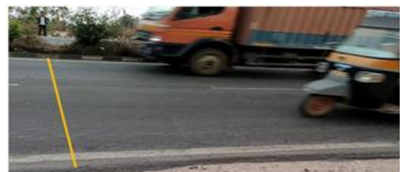
Fig-4: width of pavement for selected stretch
