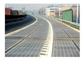
Back in 2018, China completed works on a 1- Km stretch of an expressway in Jinan. Qilu Transportation development group it consists of three distinct layers. Base layer with primary insulation, Solar cells in the middle layer and for the top layer transparent concrete was used.
