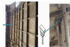
Plate 1.5.1-Beam side panel & prop head
