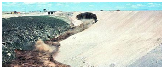
Fig -5: Photograph of Teton Dam: approaching mid-day, the leak has enlarged further and widened under the crest [5].
