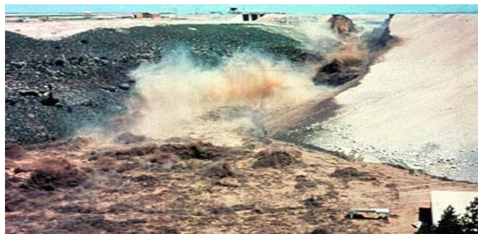
Fig -7: Photograph of Teton Dam: leak has enlarged and widened, crest (bridge) has collapsed, the outflow exceeds 28,300 m 3 /s eroded all the dam fill, [5].
