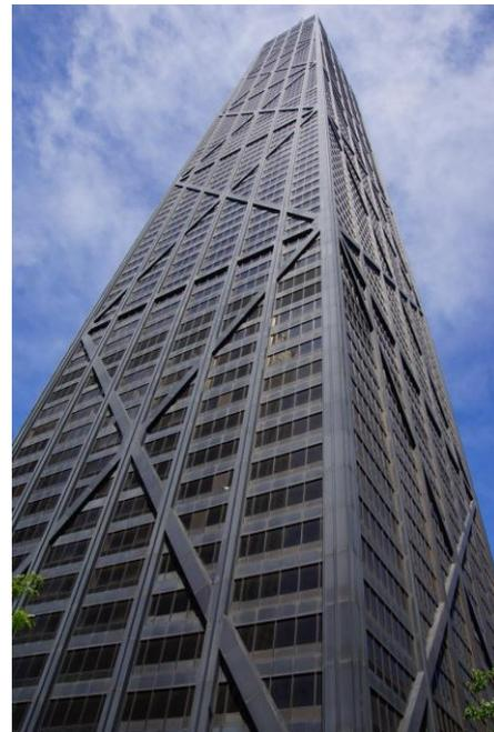
Fig. 3 Tube system in tall building.
