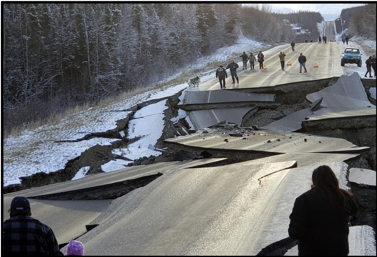
Figure 3. Damaged Highway Due To Earthquake.
