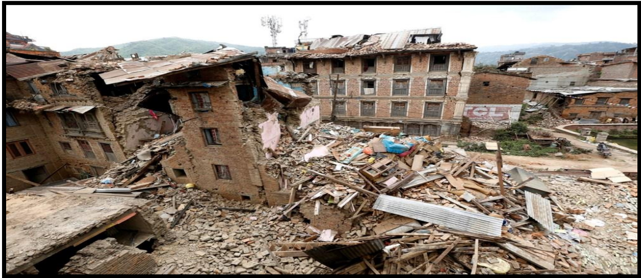
Figure 2. Damaged Infrastructure Due To Earthquake
