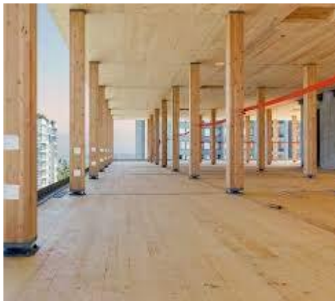
Fig -3: CLT FLOOR & ROOF
