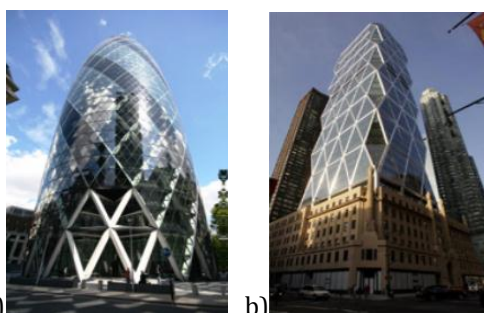
Fig-1: Diagrid structures (a) Swiss Re in London (b)Hearst Tower in New York
