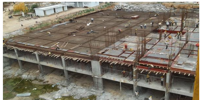
Fig. No.1 Conventional Formwork.
