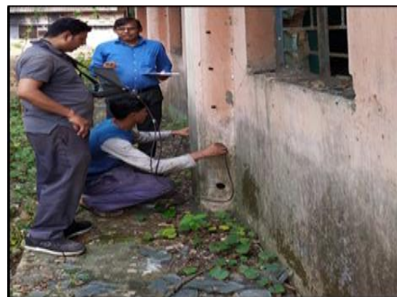
Fig: 3 UPV Test by Direct Method on Column
