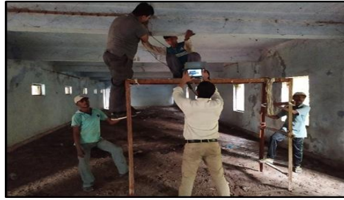
Fig: 6 UPV Test by Direct Method on RCC Beam
