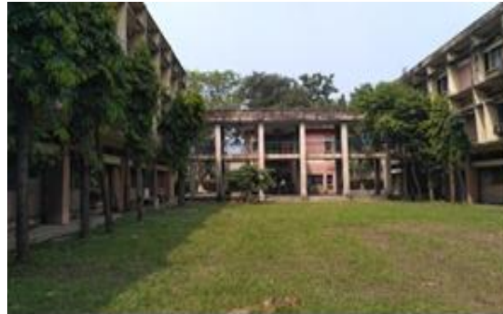
Fig: 1 View of Concrete Structure (Building)
