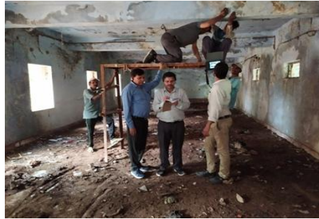
Fig: 5 UPV Test by Direct Method on RCC Beam
