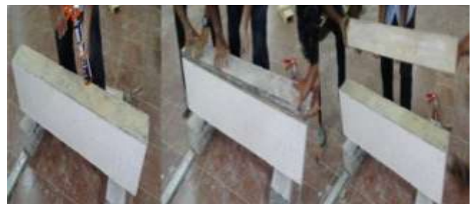
Fig -4: Attaching panel using Adhesive
