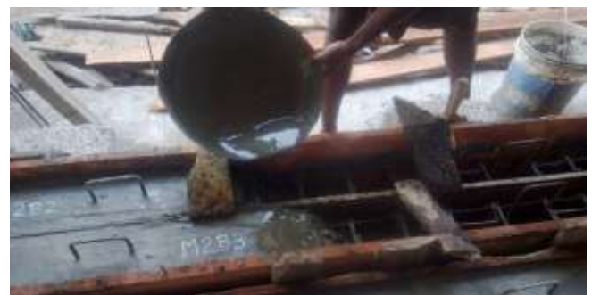
Fig -1: Cement slurry application for joint preparation in RCC beam
