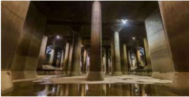
Fig.13 Metropolitan Area Outer Underground Discharge Channel
