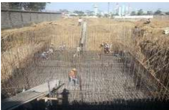
Fig.4 Construction of rectangular tank
