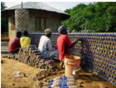
Fig -1: Placing of Bottle Wall Structure
