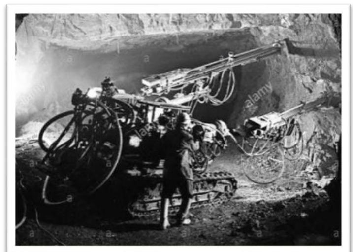
Fig.3.2. Drilling by Jumbo Drill Machine.
