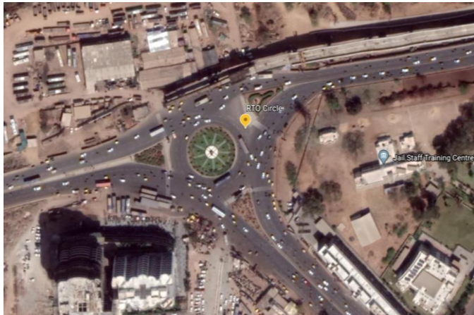
Fig -1: Aerial photograph of RTO circle
