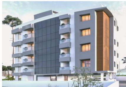
Fig 1. G+4 residential Building
