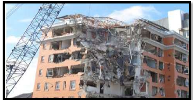
Fig.1 - Demolition of structure.
