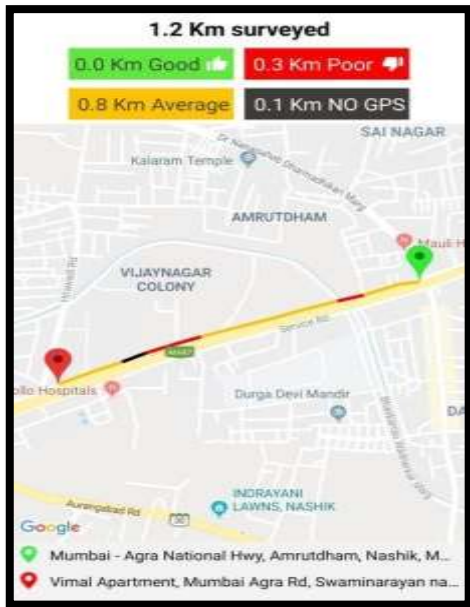
Figure 1.3: Road condition of study area by using “Road Bounce Application”
