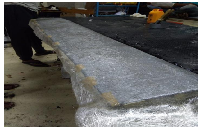
Fig -7: Apply layer of Fibre reinforced plastic.
