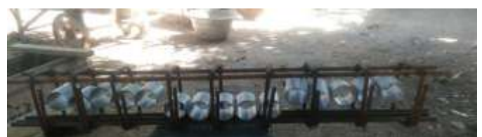
Figure 5: Arrangement of PVC pipes in longitudinal zigzag position.
