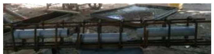
Figure 4: Arrangement of PVC pipes in longitudinal zigzag position.
