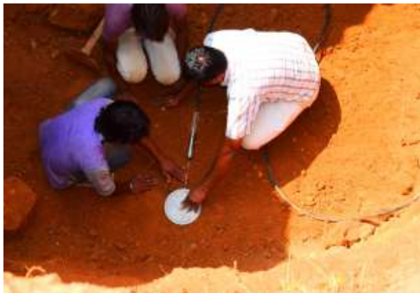
Fig -6: Pressure Cells installation
