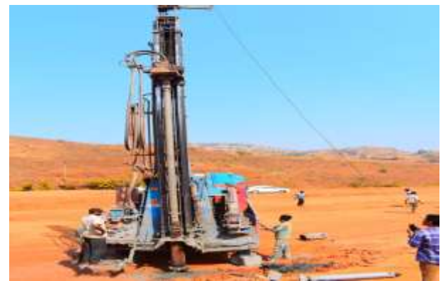
Fig -4: Vibrating Wire Piezometer installation
