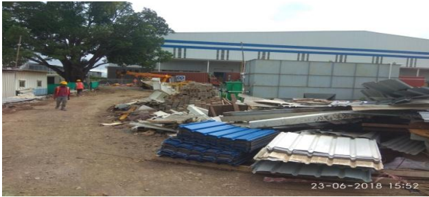
Wastage due to cutting
