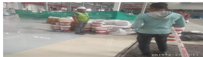
Storage of aluminum materials
