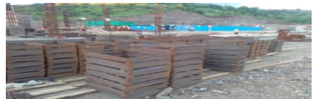
Steel must be stored on raised platform and tarpaulin covering with segregation
