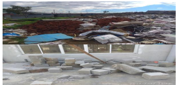
Wastage due to bad storage and cutting
