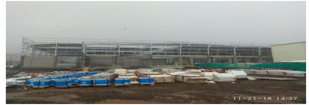
Sheeting materials to be stored near to site and on raised platform and with proper tarpaulin cover to prevent contact with soil and moisture and for less handling.
