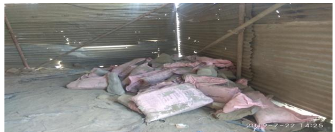
Wastage due to poor storage
