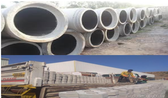
RCC pipes and grass paver to be stored on leveled ground with category wise
