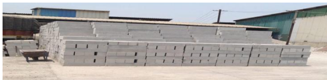
Fig.12. - Suggests ways to store bricks and blocks on construction sites.
