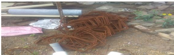
Steel remains un-used due excess order Wastage due to cutting non economical
