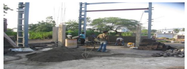
Wastage due to bad storage and cutting
