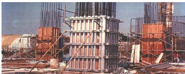
Proper stocking of timber material
