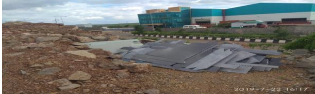
Poor methods of storing of tiles
