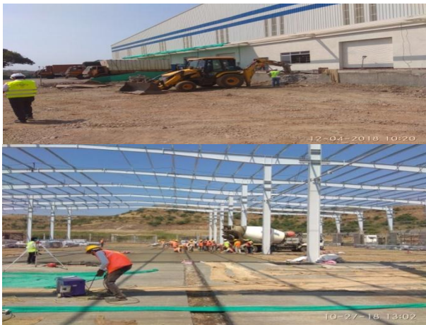
Wastage due to rework, mistake Wastage due to extra thickness of pcc
