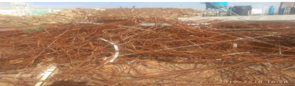
Steel remains un-used due excess order Wastage due to cutting non economical
