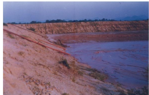
Fig -1: Stockpiles of Red Mud at a Disposal Site[4]
