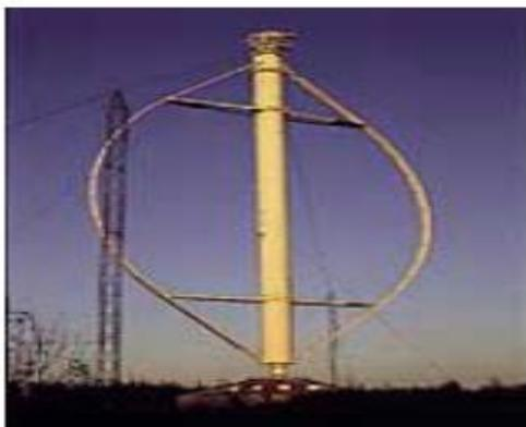
Figure1.2: Vertical axis wind turbine
