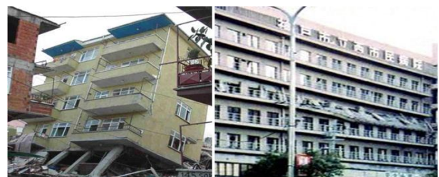
Fig -1: Soft storey collapse (Ground and intermittent storey)
