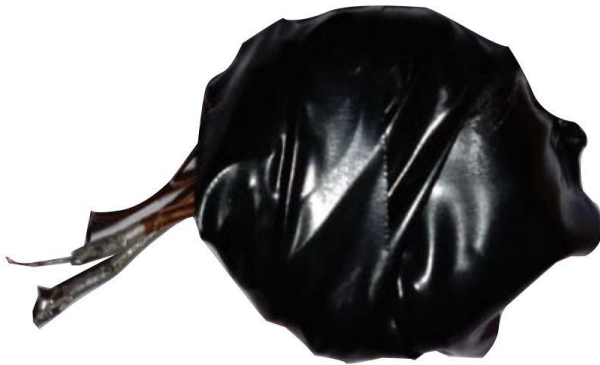
Fig -8: Current Transformer
