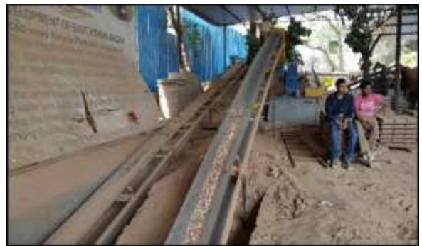
Fig -3: Feeding of waste to crusher
