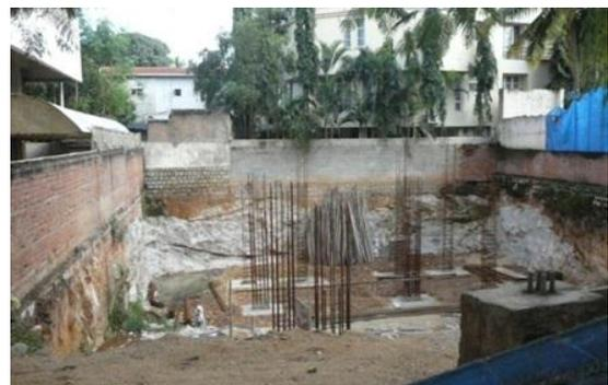
Fig -1: Deep excavation for basement
