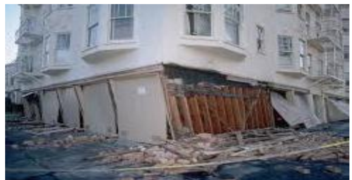
Fig-1: Typical open ground storey building
